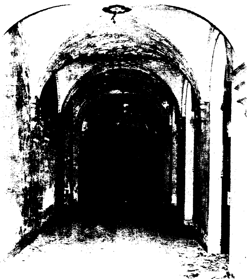
An arched hallway with sagging and peeling plaster gives a hint of the former grandeur of the mansion, which for the most part, was designed in "1930 Hollywood."
