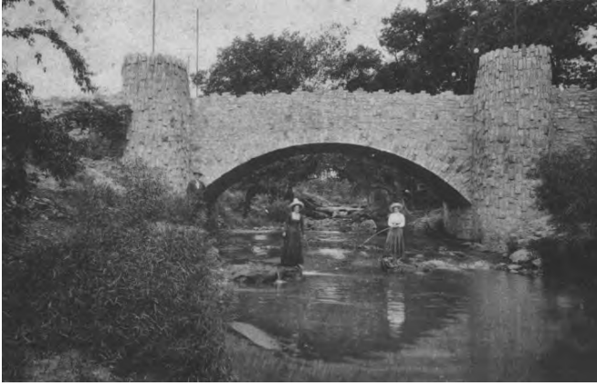
Figure 3-47. Postcard view of Lincoln Bridge, circa 1920. Note vertical and horizontal coursing in the masonry.
