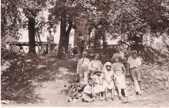
Figure 3-42. Black Sulphur Springs Pavilion under construction, 1929. Note tile outlet in foreground.
