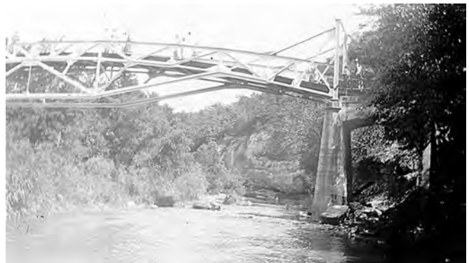
Figure 3-23. Concrete abutment for the “Rainbow Bridge,” no date.
