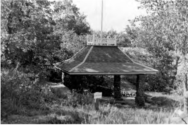
Figure 3-67. Hillside Springs, circa 1933. This photograph was taken prior to the changes made by the CCC.
