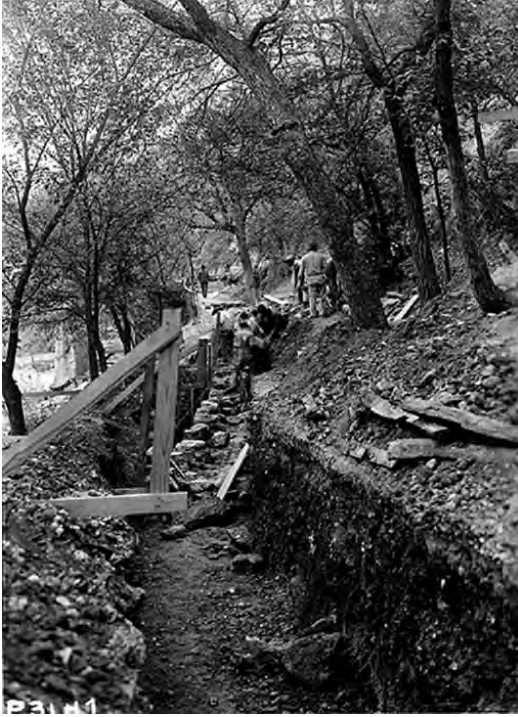
Figure 3-34. Bromide trail and wall under construction, 1931. “Before” view of Figure 3-35.
