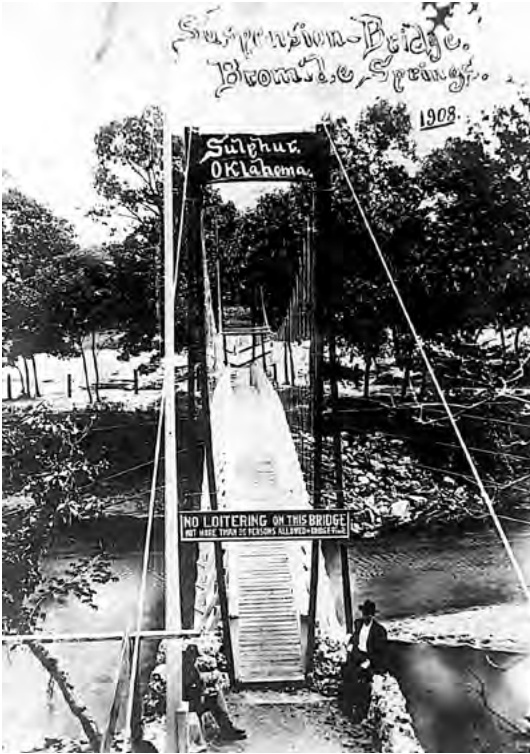
Figure 3-19. View north down the swinging bridge, 1908.
