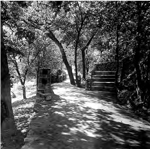
Figure 3-36. Completed Bromide trail and wall, 1932. Note difference between new masonry (left) and pre-1930 masonry (right).
