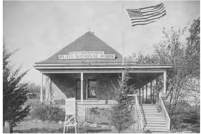
Figure 3-62. Superintendent's Office, formerly the Leeper House, circa 1918. Note weather station in foreground.
