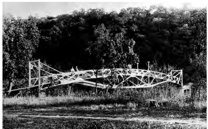
Figure 3-24. Rainbow Bridge at Bromide Springs, circa 1920. Note electric lights on span.
