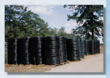
About 686 miles' worth of piping was installed in the heat exchangers at Fort Polk. The pipe was preassembled and installed as "uni-coils," so the only fusion joints in the piping are near the surface—one of several measures to control installation and maintenance costs.
