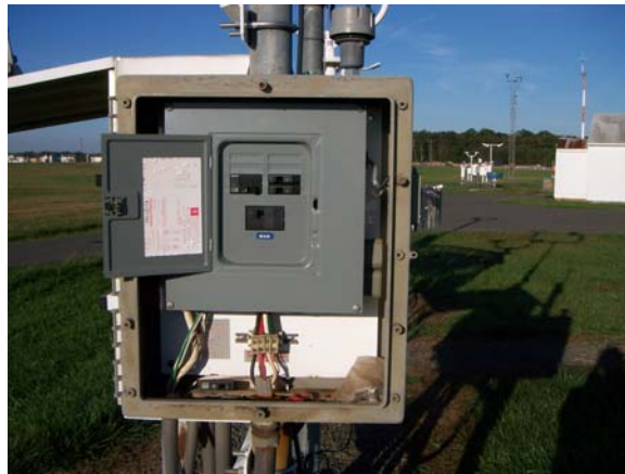
Figure 10 : Typical AC disconnect box and breaker panel
