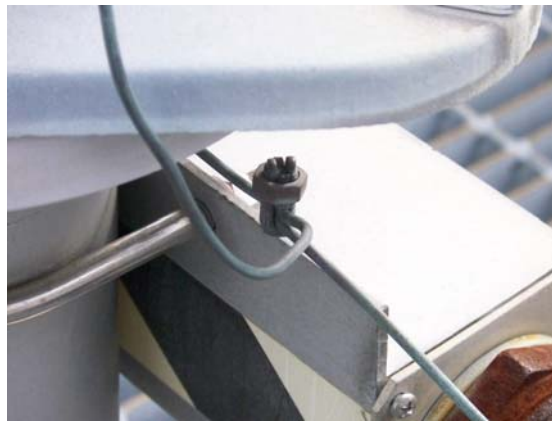
Figure 13 : Ground connector installation
