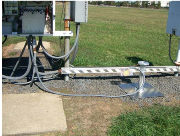
Figure 14 : Completed installation showing nylon tie wrap location
