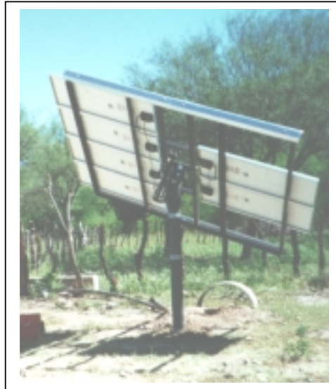
Figure 4: The tracker is a pole-mounted mechanism that supports the PV array structure designed to maintain the array tilted toward the sun, thus maximizing the solar energy captured by the array and converted to electricity. It can increase water production by 20 to 30%.
