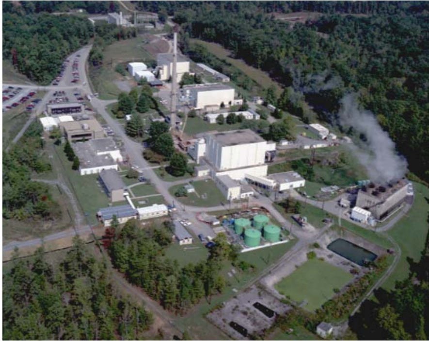
Figure 7-1. Building Complex Housing HFIR, ORNL
