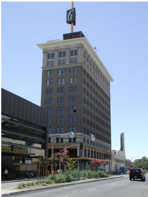
Figure 20: Guaranteed Savings Building, Fresno, CA
