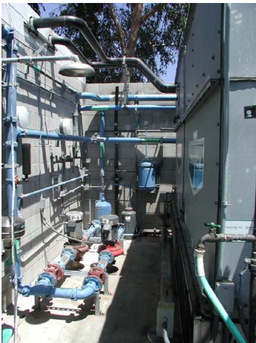
Figure A- 33: Water Heating and Cooling Loops
