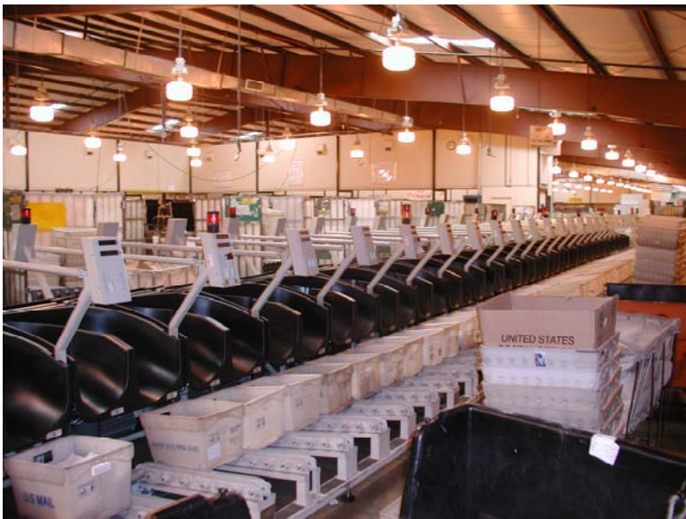
Figure A- 36: San Bernardino mail handling equipment (annex space)
