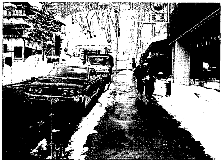
Figure 3. Jozankei Chuo Road embedding snow melting system. No snow is seen on carriage way and sidewalk.
