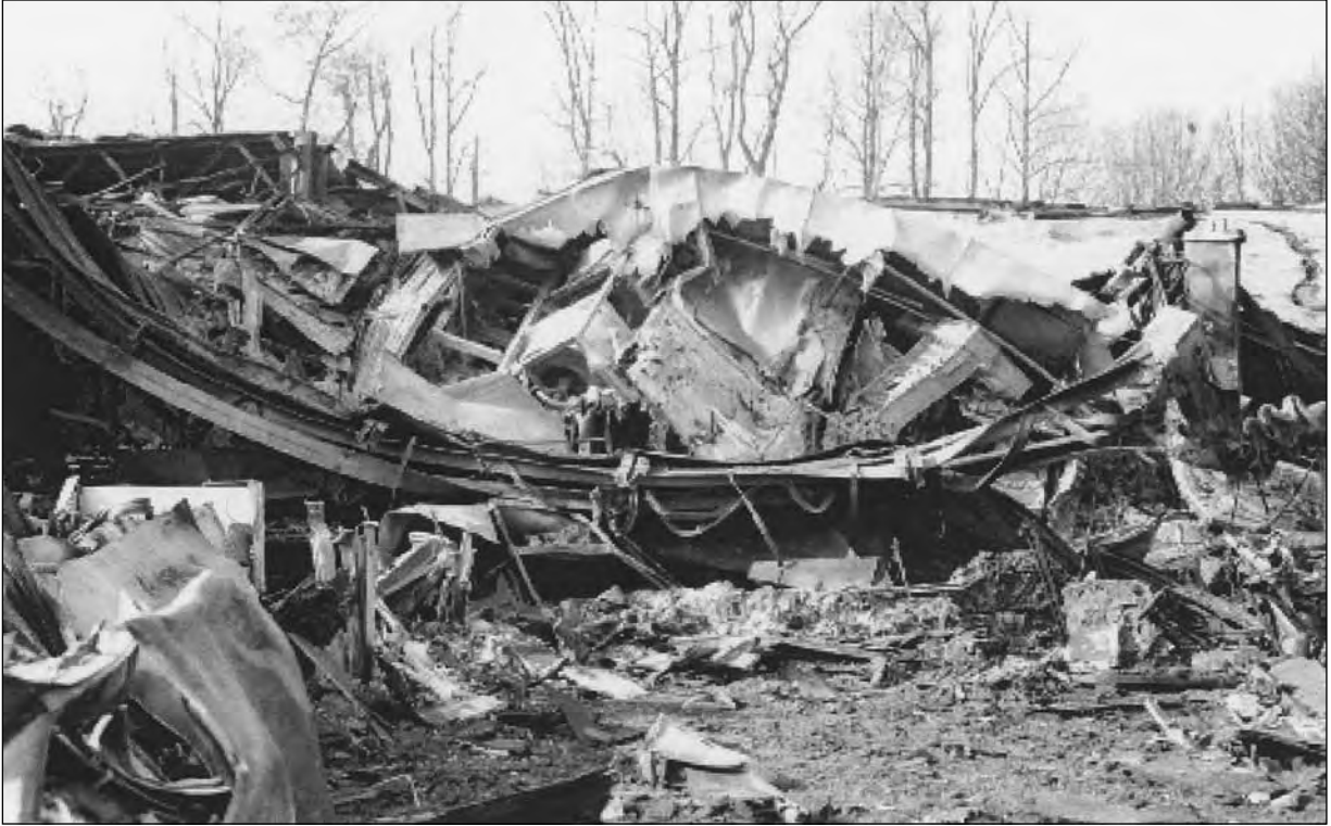
Figure 9. HVAC unit (arrow in Figure 5) after fire, viewed from northeast.
