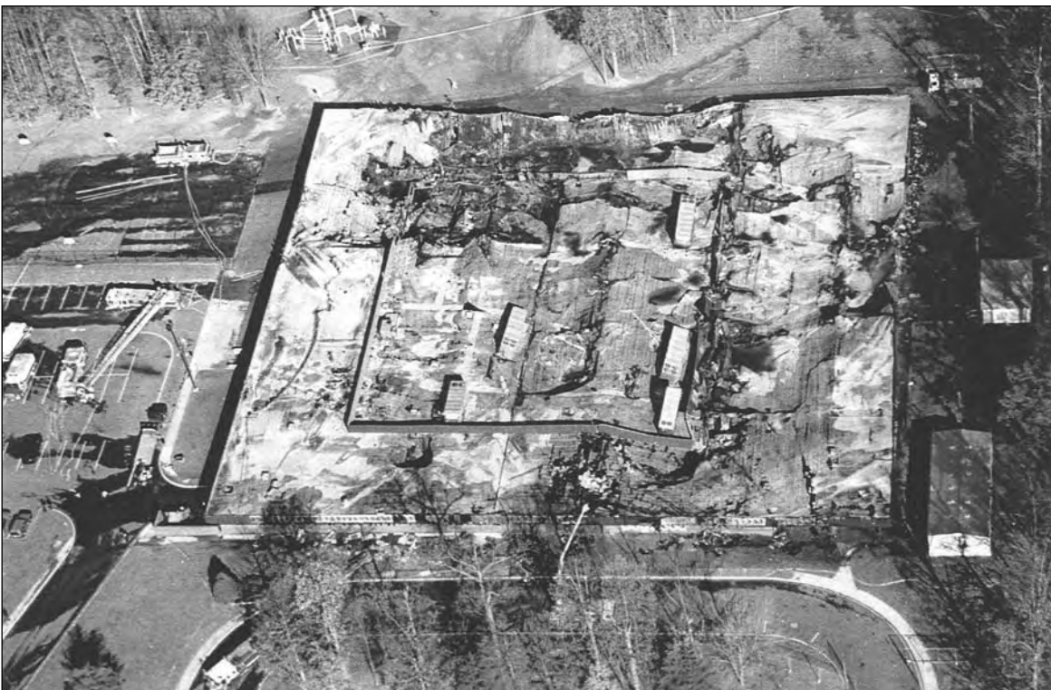
Figure 6. Aerial view of Dogwood Elementary School after the fire.
