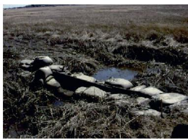
Figure 11. Ditch plug in an OMWM system.
