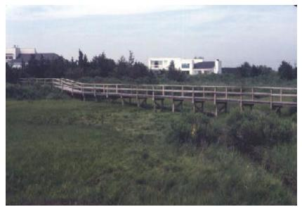
Figure 10. Walkway to a dock constructed over salt marsh.
