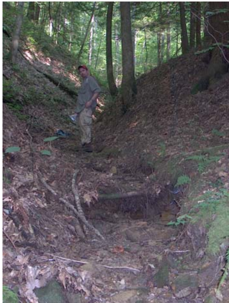
Figure 3-14 Subtle headcut in Falling Rock Creek in east-central KY (looking upstream).
