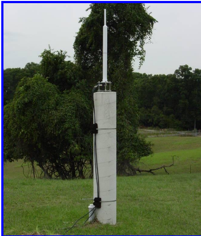
Figure 4. DORIS GREB antenna on the pillar monument
