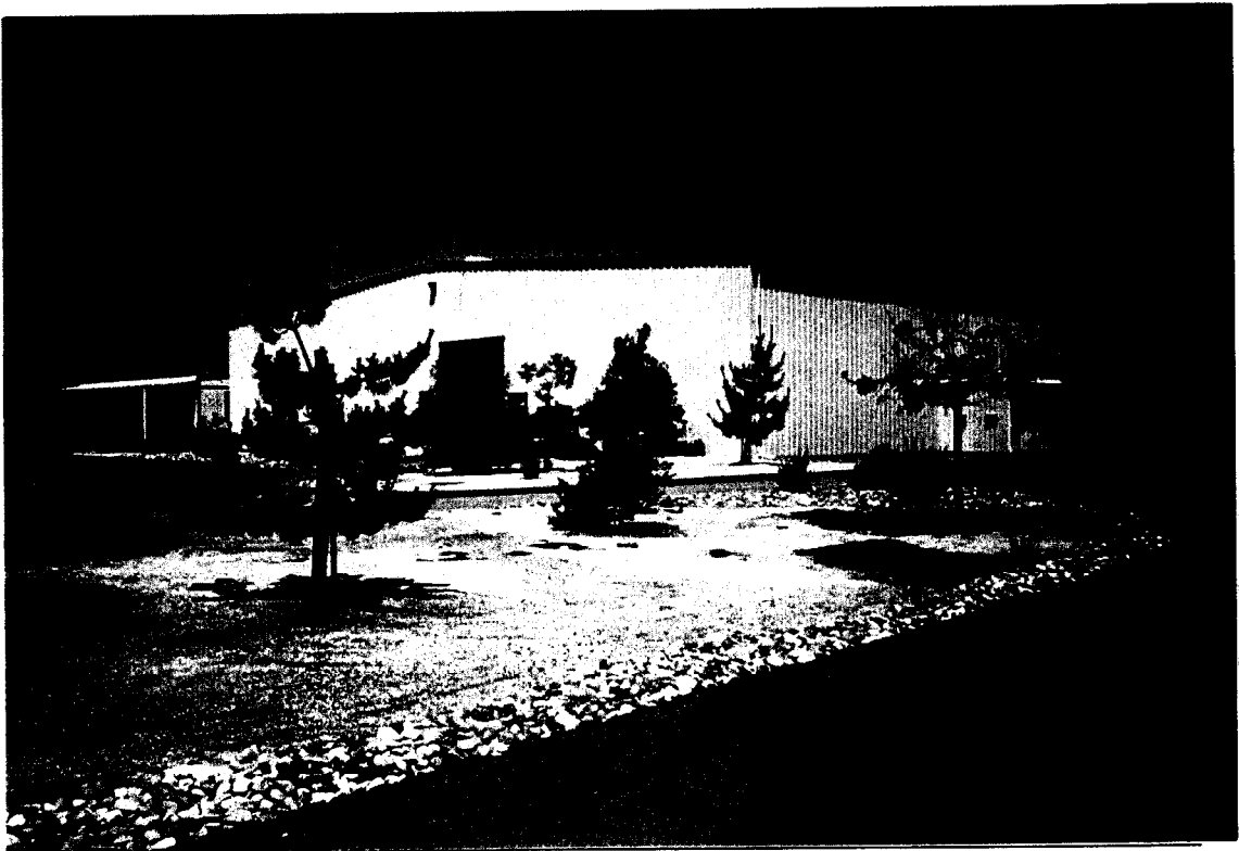
Photo 1: Groundwater Treatment Plant Building
