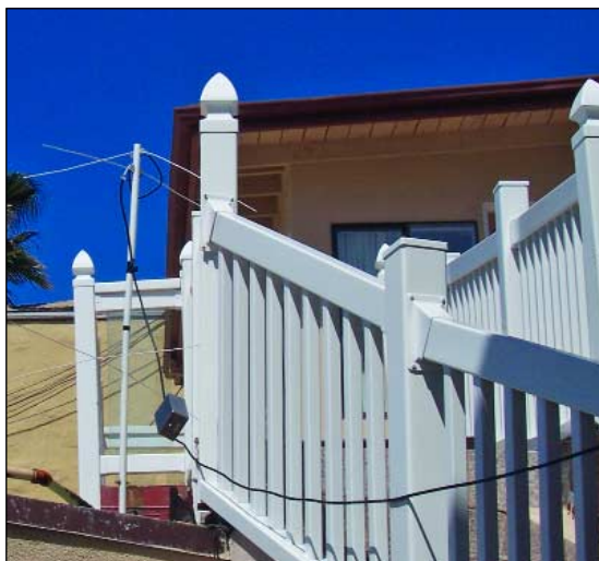
Figure 5 Turnstile Antenna located on a Hotel Stairway in Lagfuna Beach, USA.
