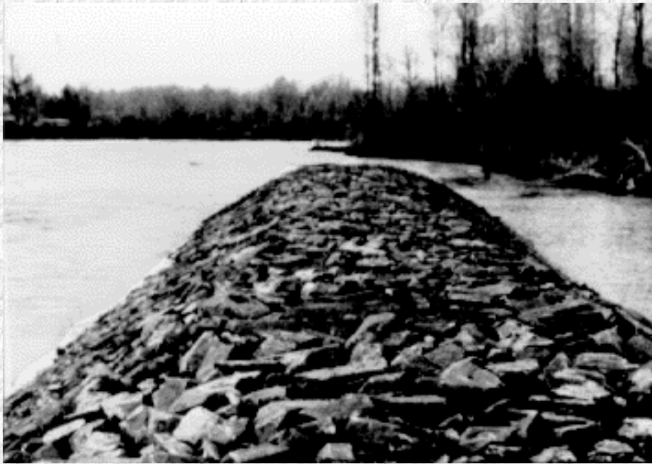
Figure 7. Plated or Keyed Riprap
