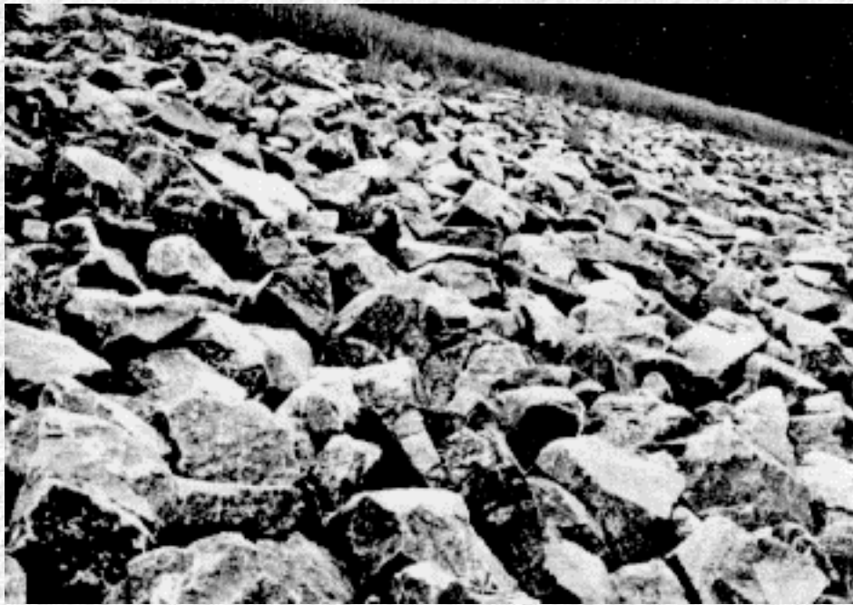
Figure 5. Dumped Rock Riprap
