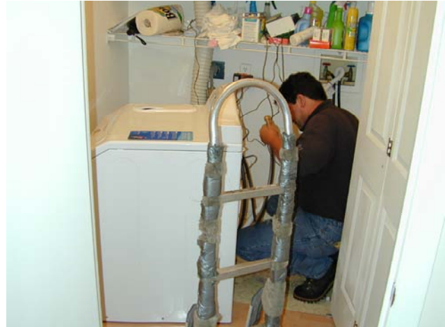
Figure 2.6 Phase II Instrumentation Installation
