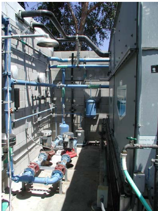
Figure A- 33: Water Heating and Cooling Loops
