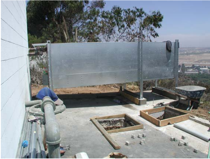
Figure A- 34: Site for the Two 150 kW Natural Gas Engines with Excess Heat Radiator in Background
