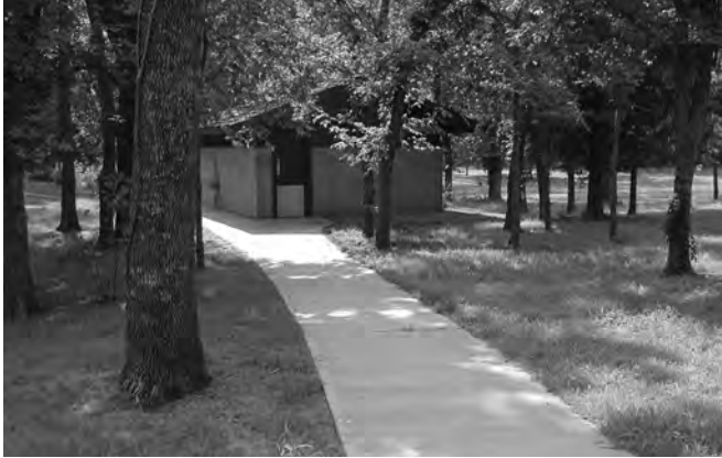
Figure 6-29. Modern comfort station and new concrete walkway, 2002.
