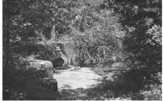
Figure 6-51. Vegetation encroaching Hillside Springs, 2001.
