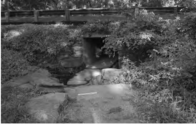
Figure 6-50. Highway 177 underpass at Pavilion Springs, 2001.
