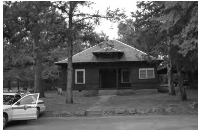
Figure 6-22. Bromide Ranger Station, 2001. Note carport on the right.
