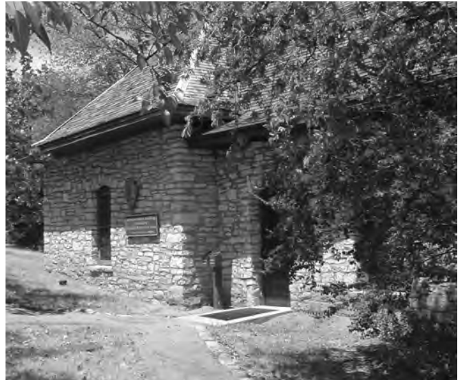
Figure 6-56. Former Administration Building (Leeper House), showing its pedestrian access, 2001.
