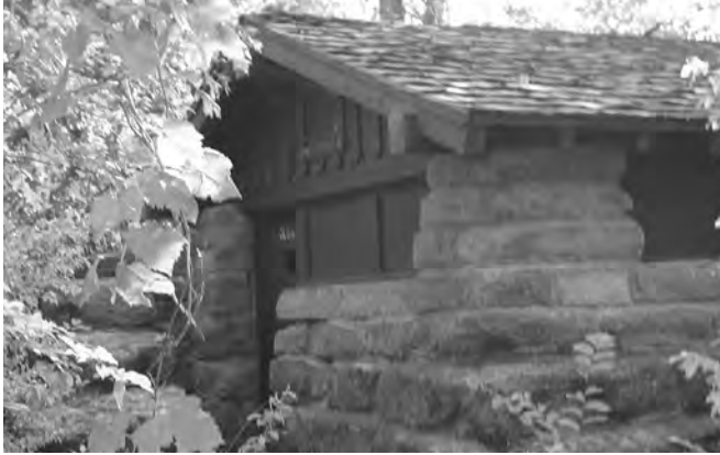
Figure 6-79. Rustic comfort station at Buffalo Spring, currently unused, 2001.
