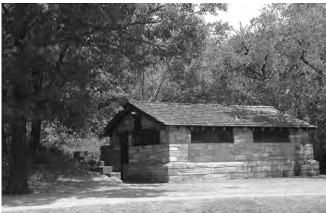
Figure 6-38. Flower Park comfort station, 2001. Photo was taken prior to 2004 pathway restoration.
