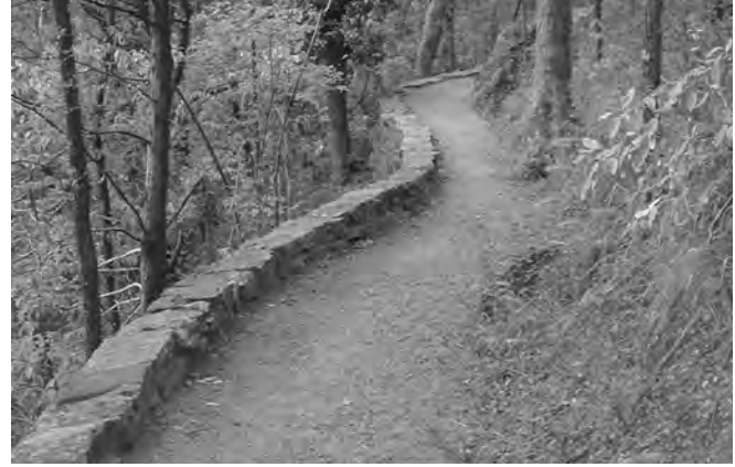
Figure 6-15. Bromide Hill Trail with retaining wall, 2001.
