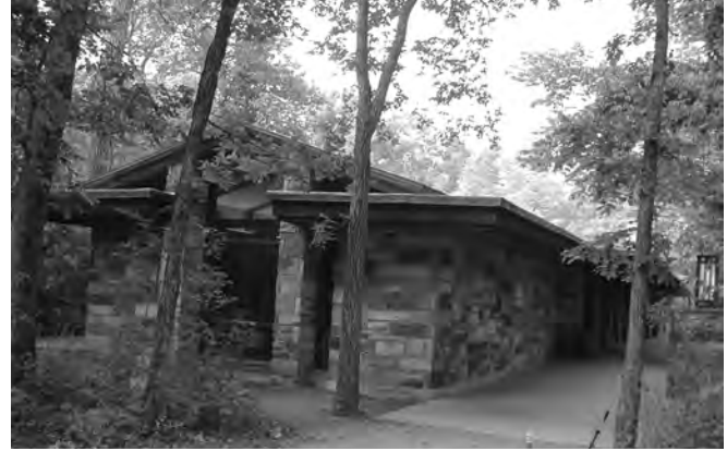
Figure 6-80. Travertine Nature Center, east facade, 2002.
