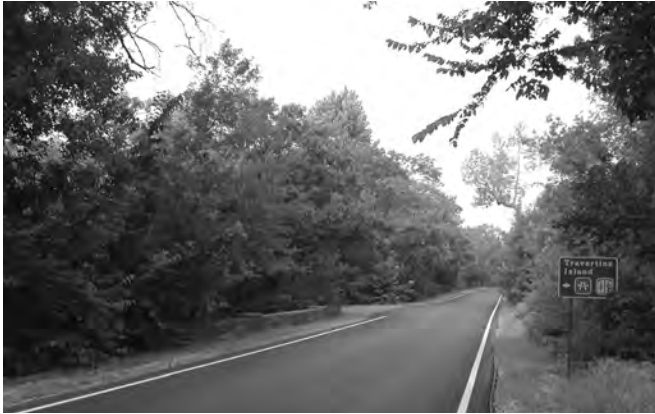
Figure 6-10. One way portion of perimeter road on Travertine Island, 2002.
