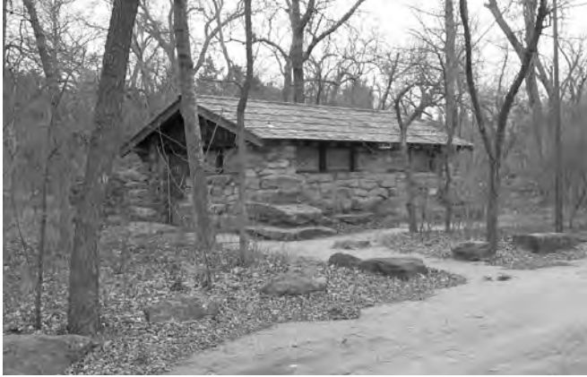
Figure 6-70. Typical Cold Springs comfort station, 2003.
