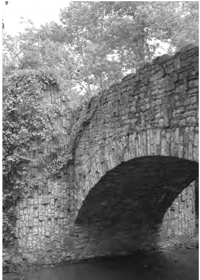
Figure 6-39. Lincoln Bridge, from Travertine Creek, 2001.
