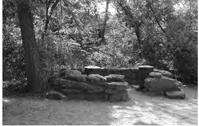
Figure 6-71. Historic wood and trash can holder typical at Cold Springs Campground, 2002.
