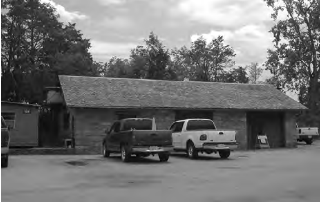
Figure 6-59. Crew room on south side of quadrangle, 2001.
