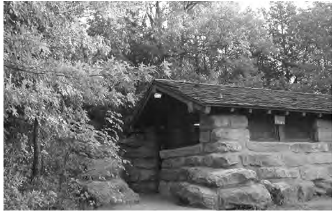
Figure 6-67. Central Campground comfort station, 2001.
