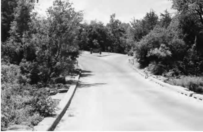
Figure 6-12. Rock Creek Causeway, 2001
