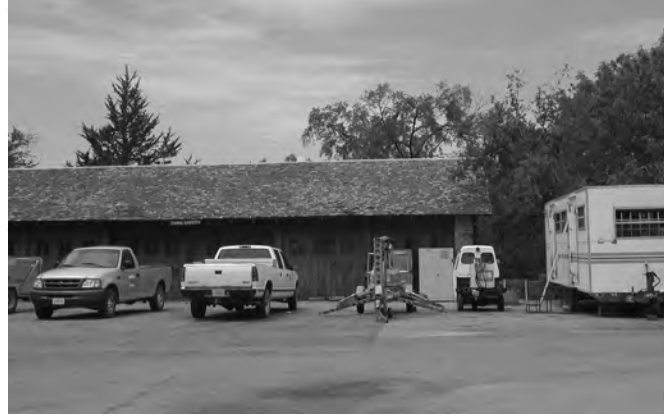
Figure 6-60 Maintenance Shop with vehicles parked in front, 2001.
