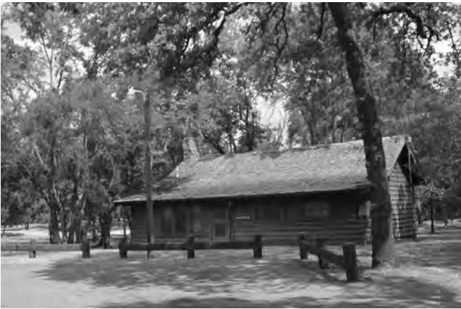
Figure 6-21. Travertine Ranger Station, 2001. Wood guardrail in front of the structure is not historic.
