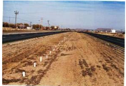
Figure 4: The planting on the median of NM Highway 124 in Milan (November 2000)
