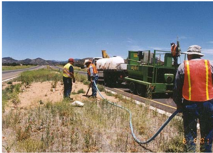
Figure 8: Applying starch-based superabsorbant to plants on the median of Highway 285 (June 2001)
