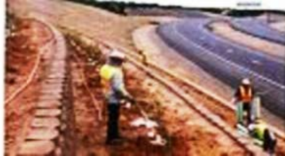
Figure 2: Watering plants through irrigation tubes to hydrate the soil in the root zone (November 2000)
