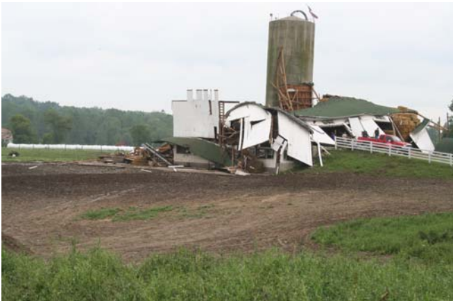
Medina Tornado Damage August 9th, 2007 NWS photo
