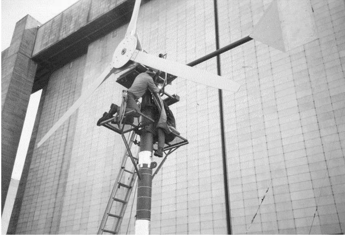
Figure 5. View of rotor outside Hangar 2 door. The rotor is mounted to the generator shaft with aluminum compression plates. The turbine is completely furled in this view with the tail angle at 90°. Bill Sorich and Jim Sencenbaugh are installing a weight pan that can be seen above Jim's head (right). Weights were added to move the center of gravity of the turbine aft.
