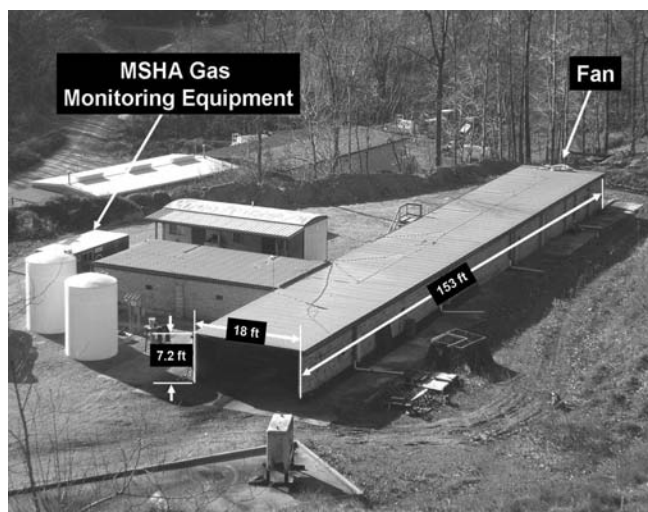
Figure 1 — Fire suppression facility.
