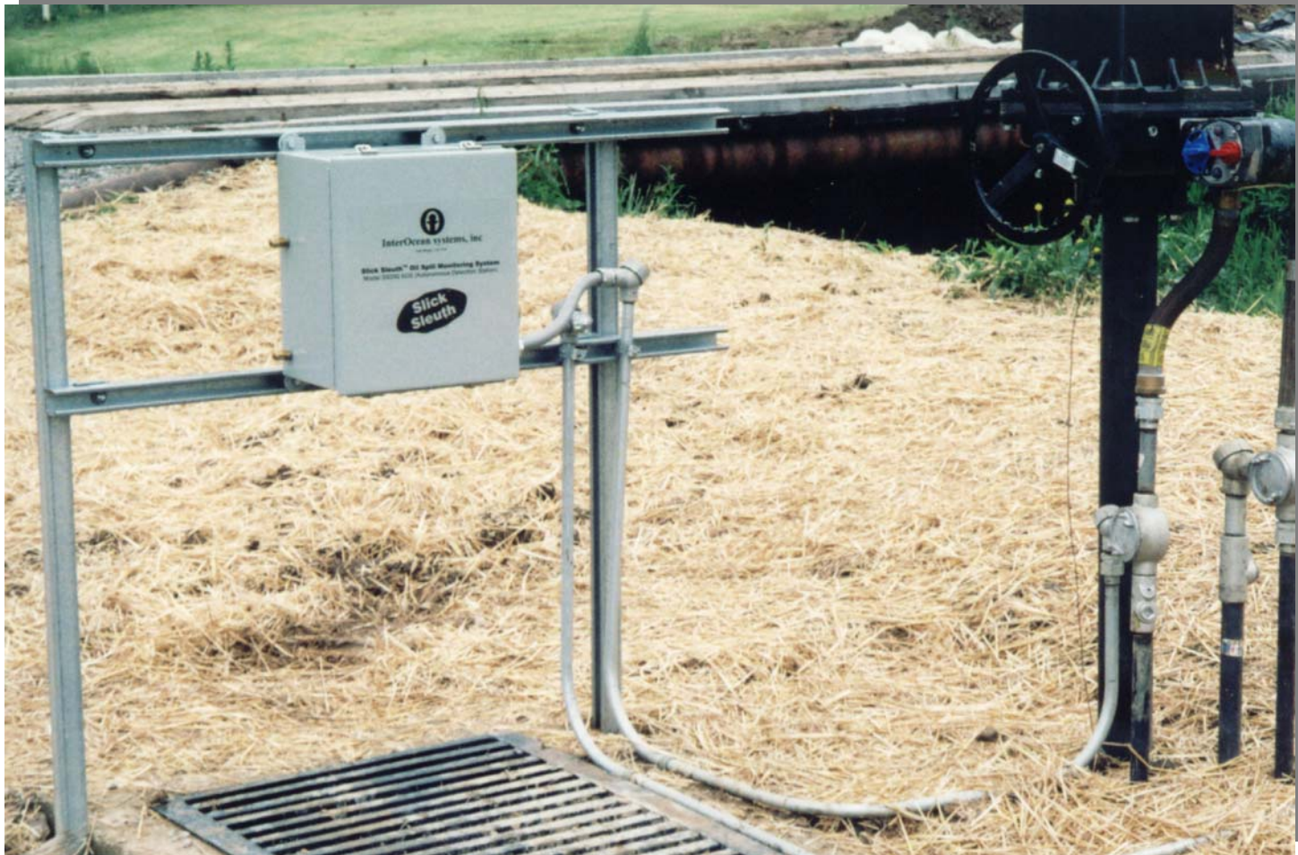
Autonomous Spill Detection Sensor w/ Actuator Valve Control & Real Time Alarm to Control Center
