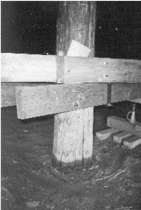
Temporary bracing supports an interior post while the concrete cures below it. Photo by David Pinyerd.
