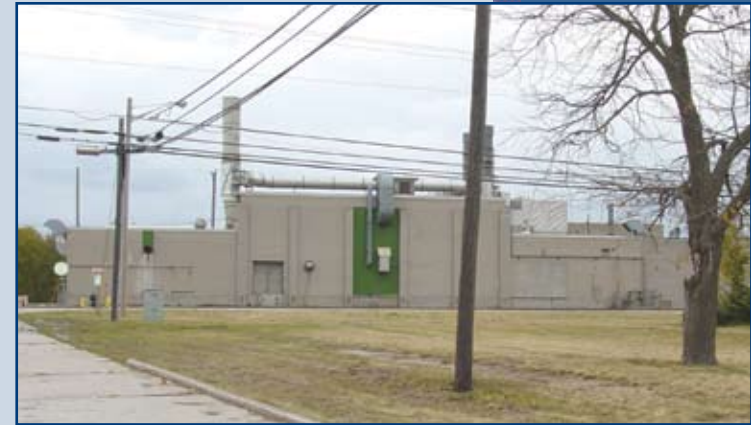
The sanctuary and local development company Alpena Marc, LLC are continuing to develop the Great Lakes Maritime Heritage Center campus. Once used for coating paper products (above), the center is now the cornerstone of redevelopment within the 29 acre historic Fletcher Paper Mill complex, located along the Thunder Bay River.
