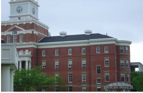
Figure 2.5 Forwood Building, US Soldiers and Airmen's Home
