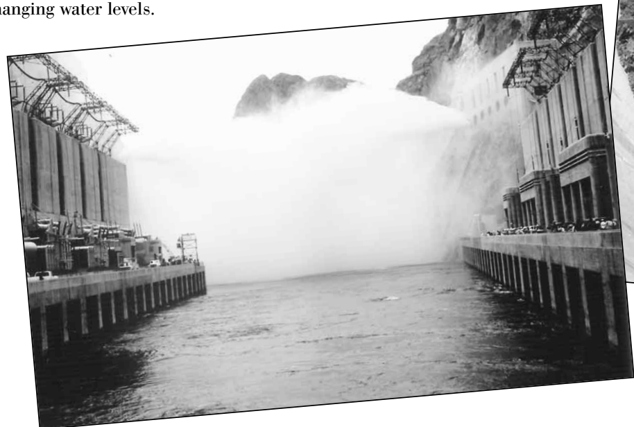
At left, the power of the release from the new jet flow gates in the upper penstock valves is captured from river level, downstream. At left and right are Hoover Dam's power plant. Photo by Steve Leon
