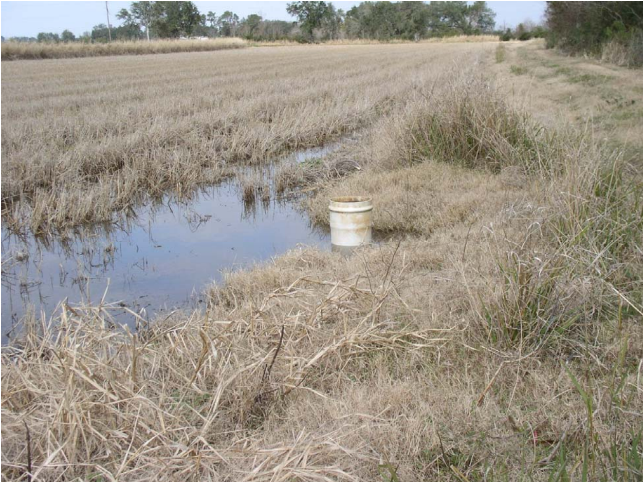
Figure 12. Grade Stabilization Structure with Riser attached
