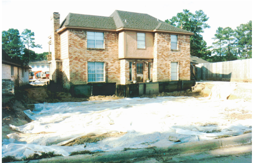
Residential Yard During Excavation
