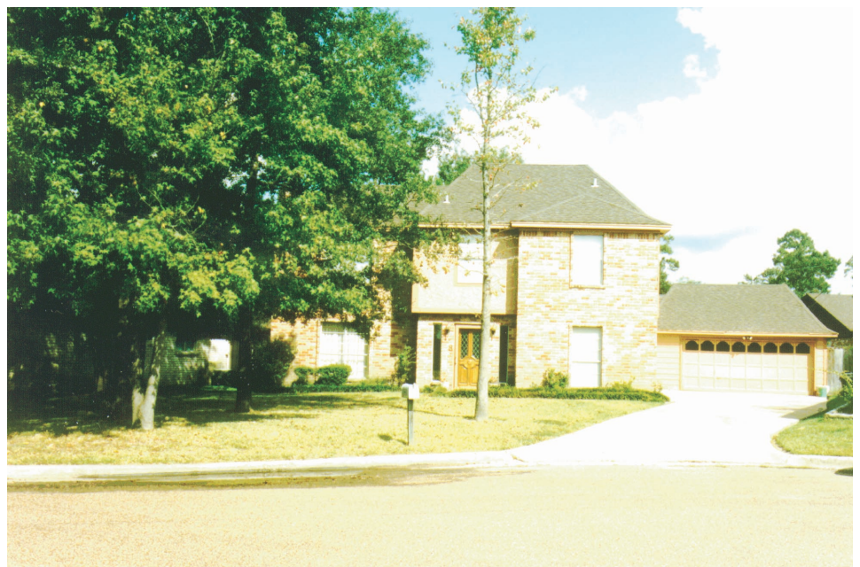
Residential Yard Before Excavation
