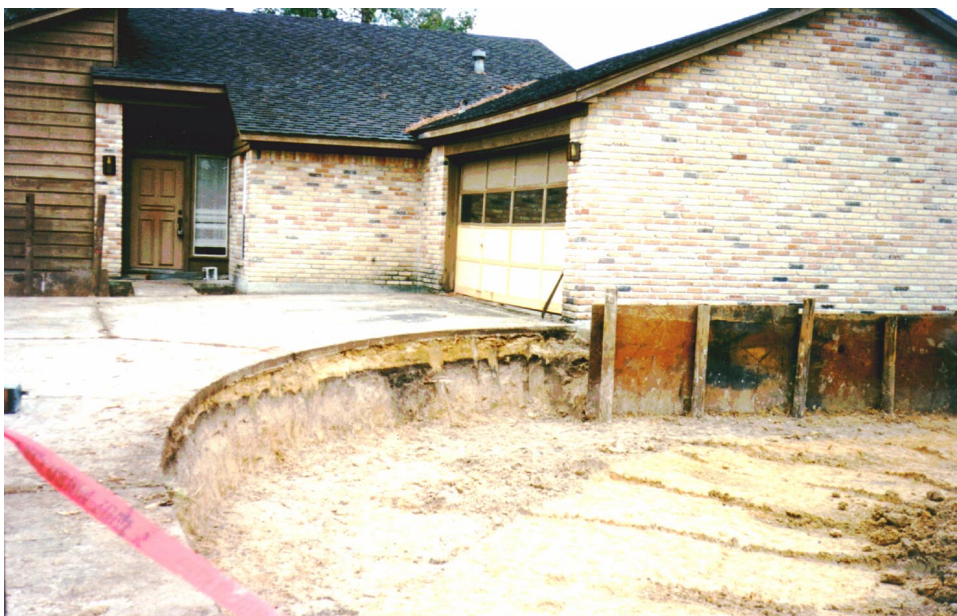
Excavation levels went to depths of five feet.
