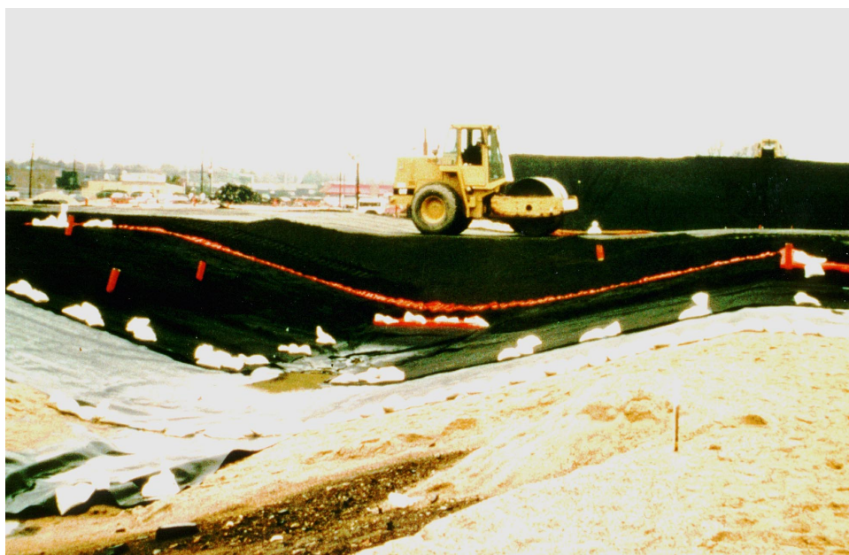
Figure 5: Construction of the Raymark Cap
