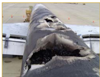
The aftermath of a cargo fire, from Class B Cargo Compartments
