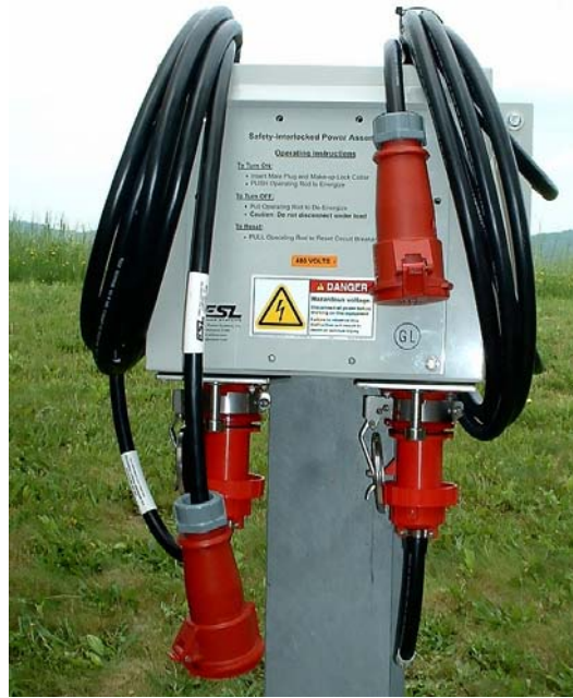
Figure 2-11: Two-Gang I-beam mounted electric connection assembly
