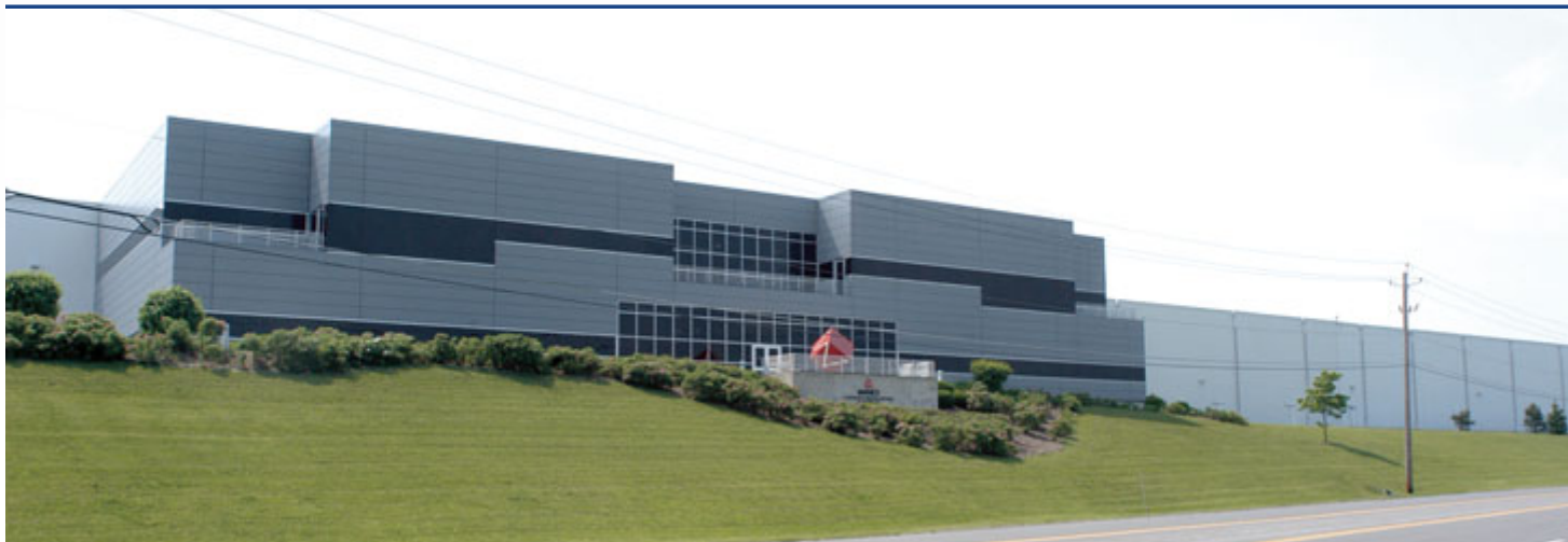
Maines’ flagship distribution center in Conklin, N.Y
