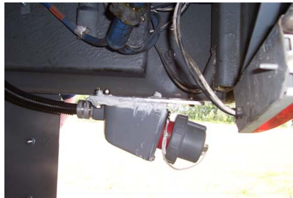
Figure 5-7. Underside View of New Trailer Plug Assembly
