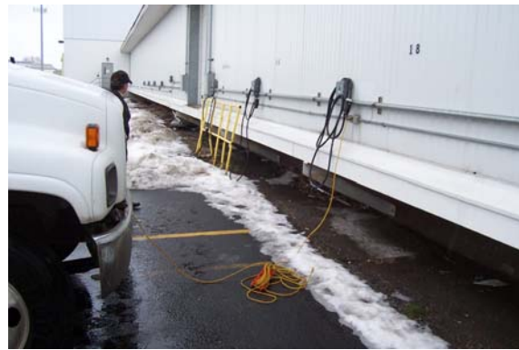
Figure 1-2: Refrigerated Box Truck Connected to Electric Power
