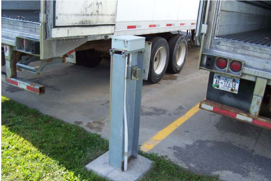
Figure 2-2: Close up of Pre-Existing I-Beam Mounts at MAINES
