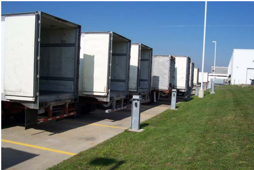
Figure 2-1: Pre-Existing I-Beam Mounts at MAINES
