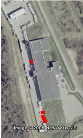
Figure 2-4: Overhead view of MAINES Facility (googlemaps.com)
