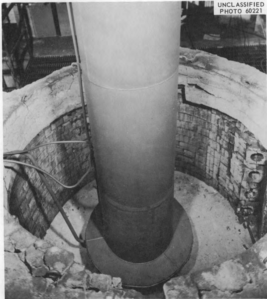
Fig. 14. Retort Top in Place for Seal Welding.
