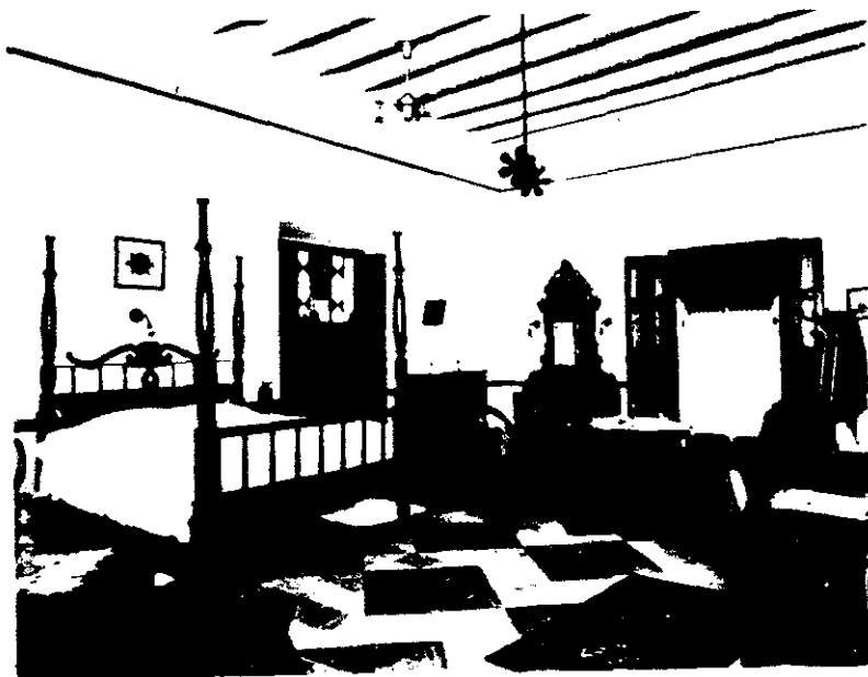
Bedroom in La Fortaleza showing type of ceiling construction being replaced with reinforced concrete
