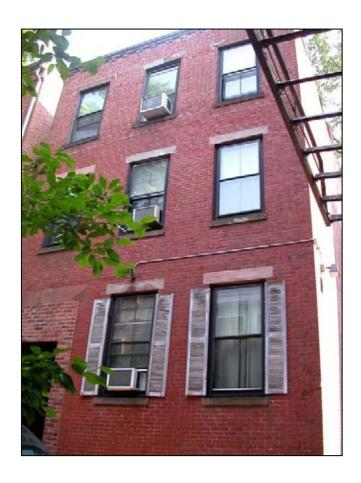
2 Smith Court is a vernacular Federal three-story, three-bay brick structure constructed in 1853. Originally constructed as a two-story structure, the third story was added at a later date.<sup>2</sup> The sidehall entry was bricked in at an unknown time to make a smaller entry. Brownstone lintels and sills frame the double-hung 2/2-light windows. At the cornice, a dog-tooth course has been used as a decorative treatment. A six-step run leads to the entry door.
