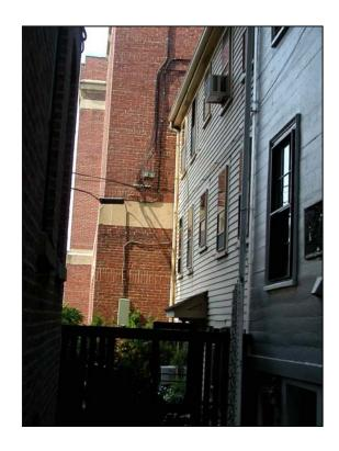
7A Smith Court is a vernacular Federal three-story, five-bay clapboard-covered structure constructed in 1799 that is located on Holmes Alley. The center entry has an Italianate-period hood added at a later date and a one-step run up to the building. Wood frames, splayed lintels, and flat sills frame the 6/6-light windows. In addition, wood shutters frame the windows on the first story. The windows over the door entry are smaller than the remaining windows. The structure has a brick foundation.
