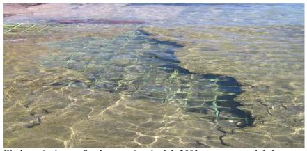
Washouts in the new South ramp after the July 2003 concrete pour left the reinforcing steel exposed. (Photo Courtesy of the Department of Planning and Natural Resources)
