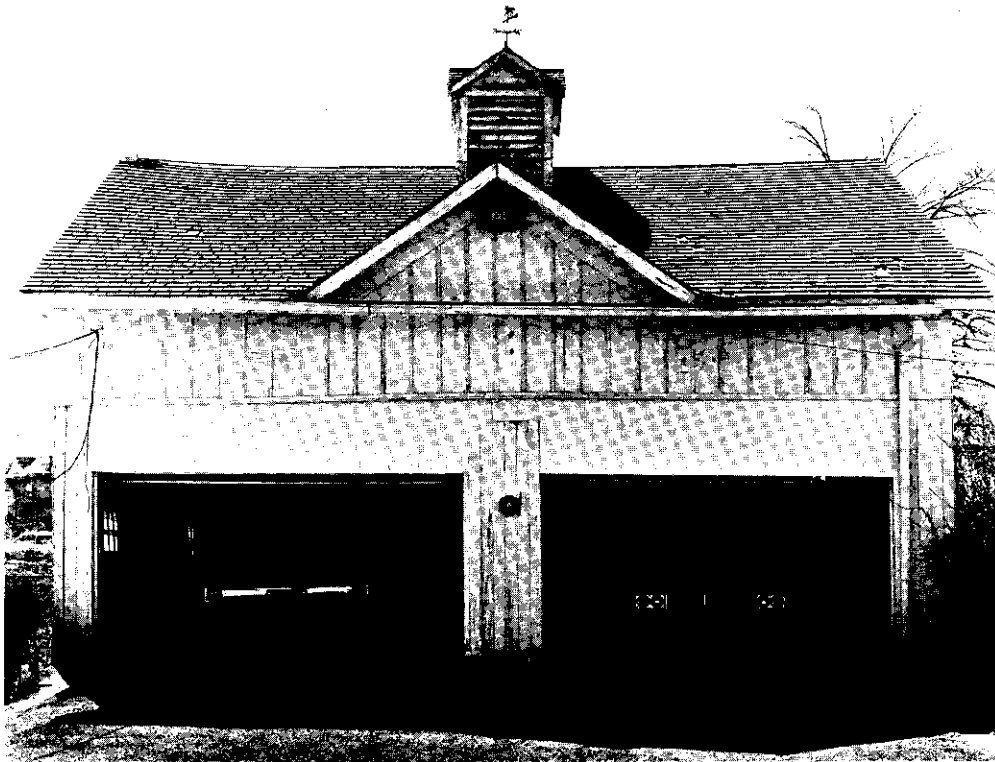
Fig. 3.1 Truman Carriage House, Fall 1985. North elevation (looking south). Credit: Zoom Studios
