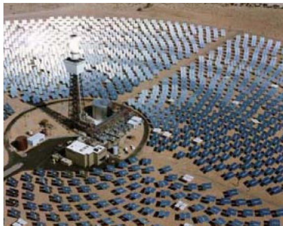
Figure 1.10. Power Tower System
