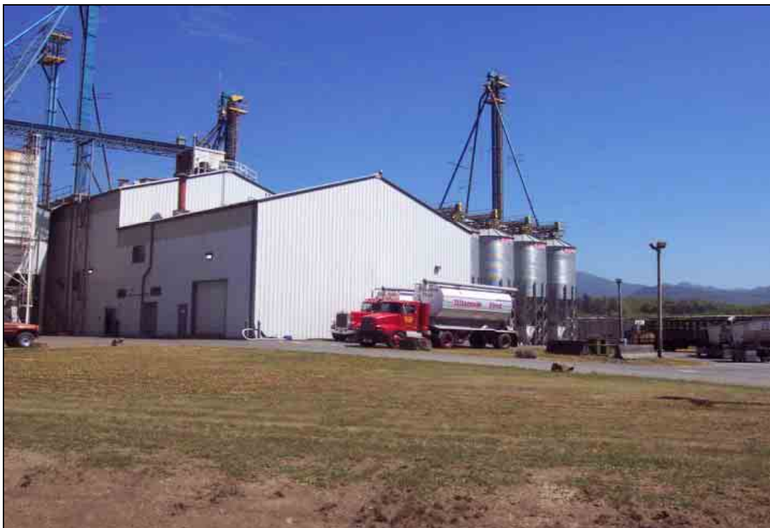
Figure C-10 Feed Mill at POTB Industrial Park – Adjacent to the Proposed Project Site
