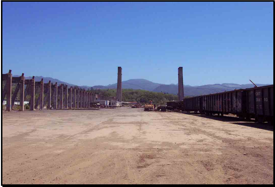
Figure 5. Concrete Pad Proposed to Serve as the Foundation for the POTB Dairy Digester & Compost Facility (Southeast Direction)
