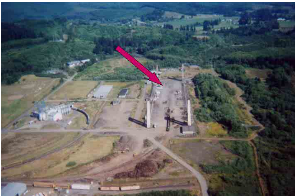
Figure 2. Aerial View of the 7.5-Acre Concrete Pad for the POTB Dairy Digester Site
