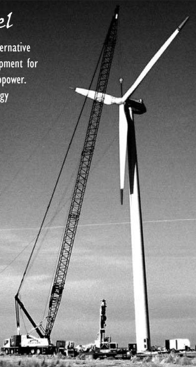
Wind turbine construction at the Rosebud Sioux Tribal Reservation in 2003.
