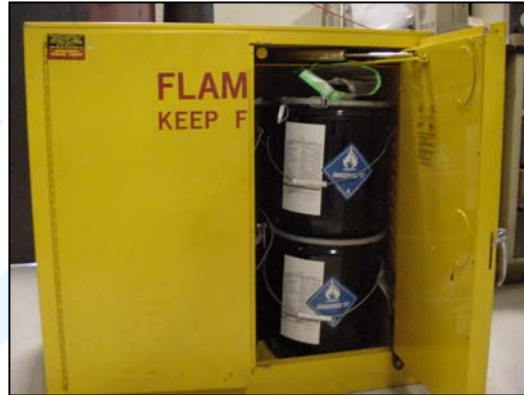
Incoming material stored in fire cabinet
