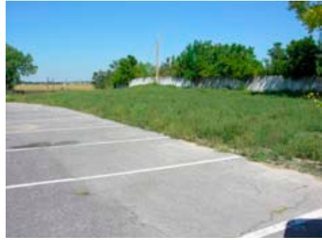
Rawhide Creek rest area along U.S. 26 near Torrington.
