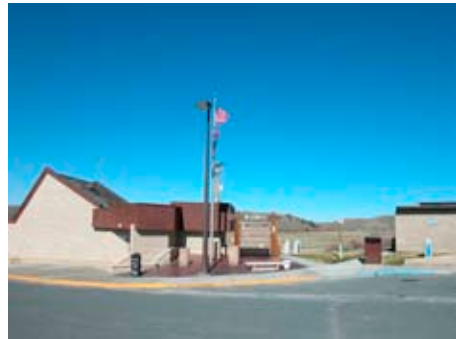
Information facility at the rest area along state road 28.
