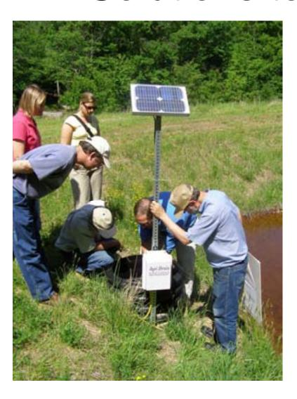
A solar powered back flush valve was installed for the pond treating seep LR0-D10.
