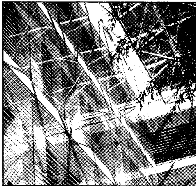
Fig. 7. Example of fritted glass curtain wall at the Federal Judiciary Building in Washington, DC.
