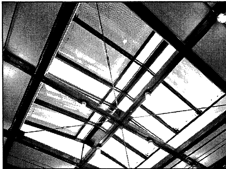
Fig. 4. PV skylight at APS facility, Fairfield, California. A standard skylight framing system mixing amorphous silicon PVs with tinted laminated glass. The PVs transmit 5% daylight.
