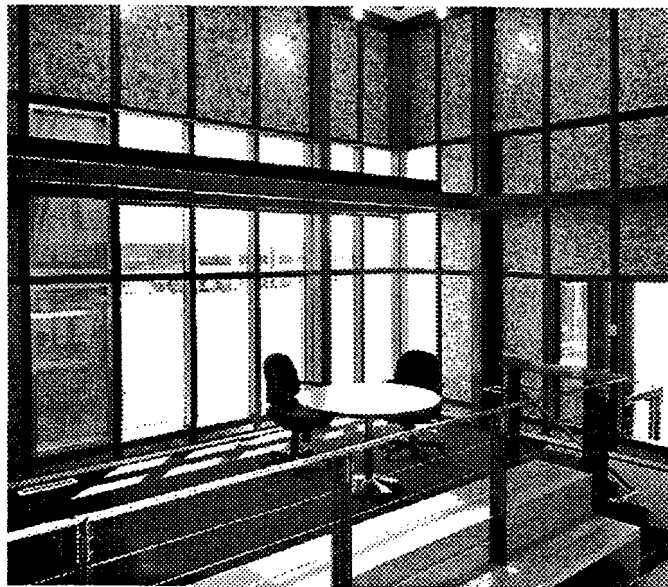
Fig. 6. Interior view of PV curtain wall at APS. For comparison, two of the PV panels to the left of the vision area are left unsealed, showing the relative transparency of the modules.
