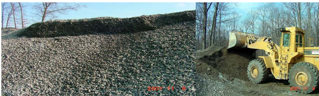
3-16 Aggregate Separation In A Pile Is Normal
