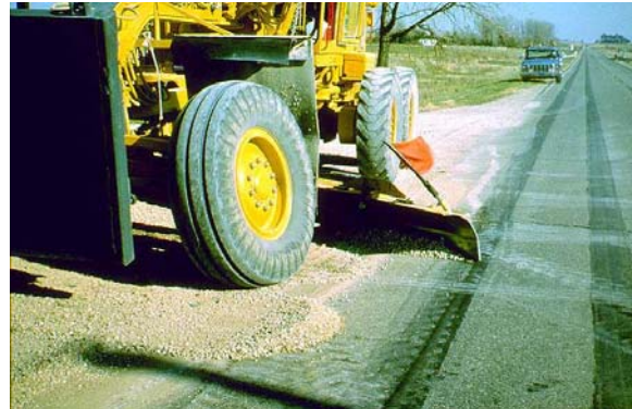
3-22 Working parallel to a paved road has advantages.
