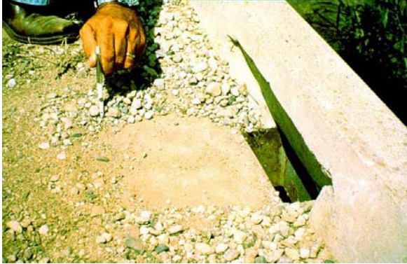
3-25 Drainage openings (scuppers) in bridge decks must be kept cleaned.
