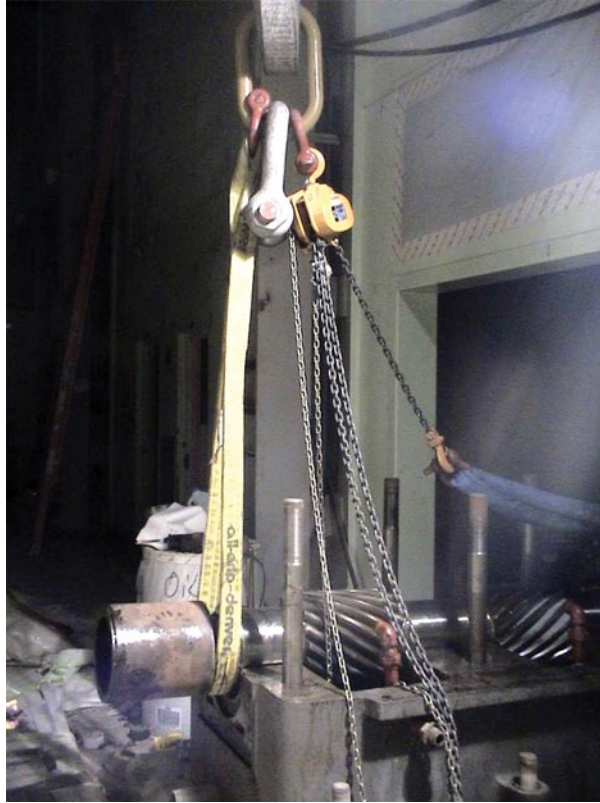
Figure 3-1. Gearbox shaft and rigging
