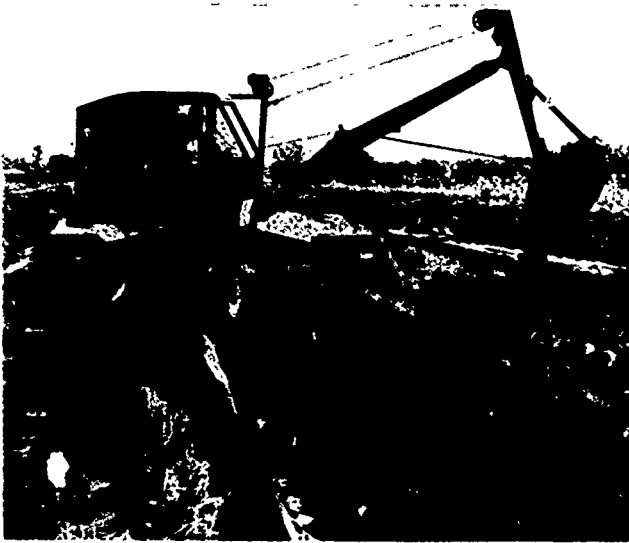
Figure 2-9—A Schield Bantam backhoe cuts new ditches in extremely wet soils on Edisto Island, South Carolina, in 1958. The wide tracks and shoes allow the machine to straddle the ditch while cleaning it.
