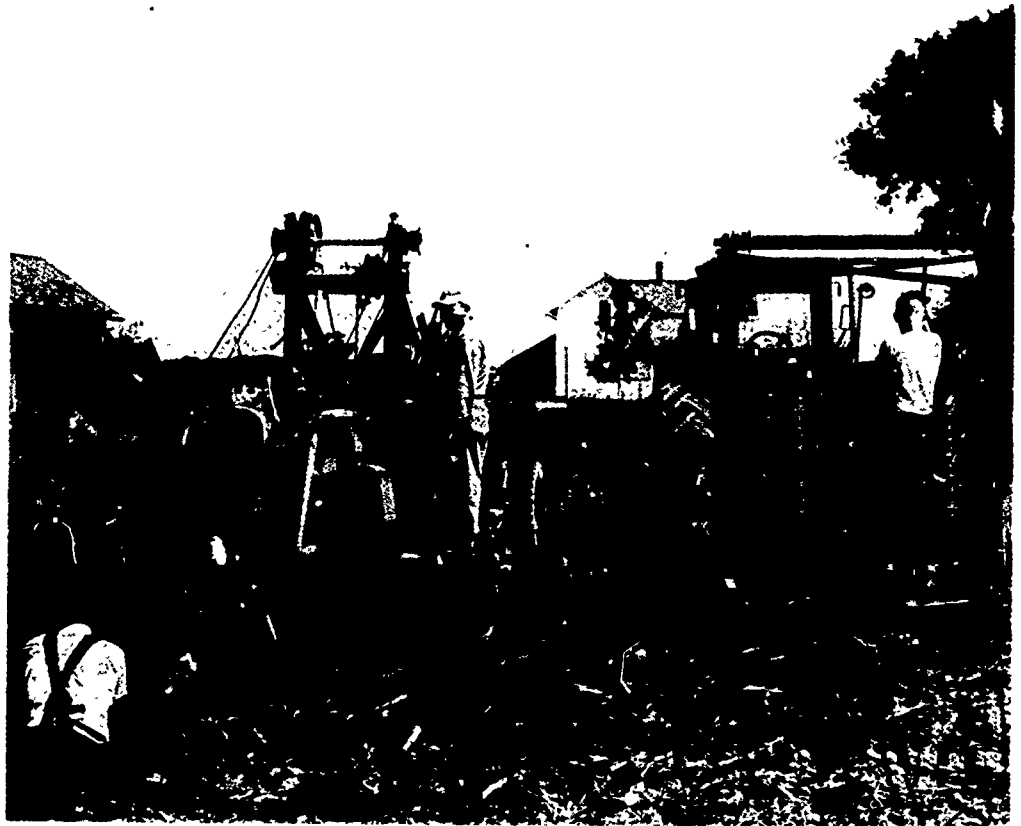
Figure 3-1—Eaton County, Michigan, workers haul palletized tile on a "chariot" connected directly to the tile machine.
