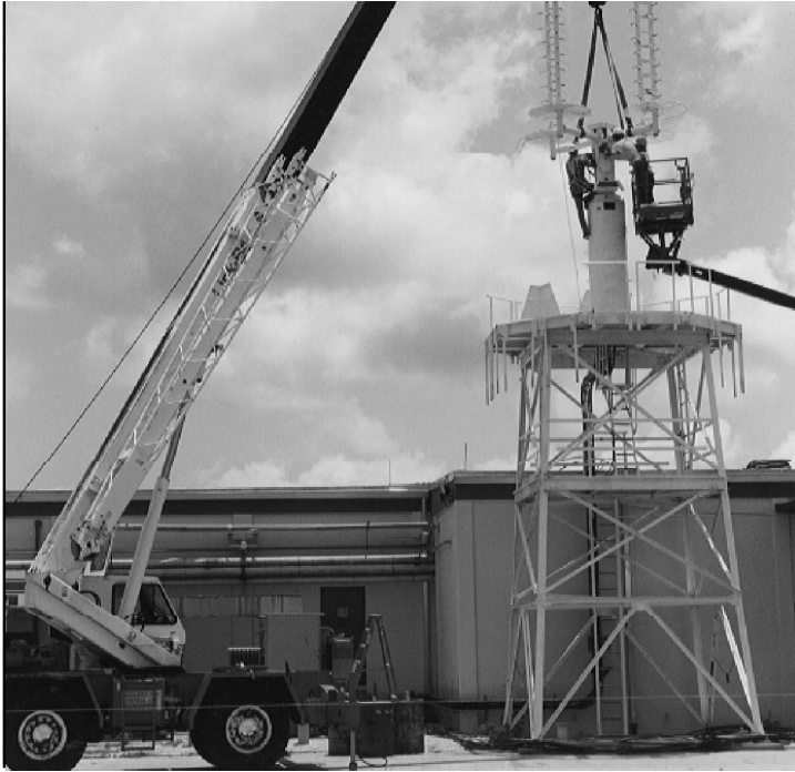
A HISTORIC tracking antenna is mounted on a pedestal at the Merritt Island Launch Area tracking station.
