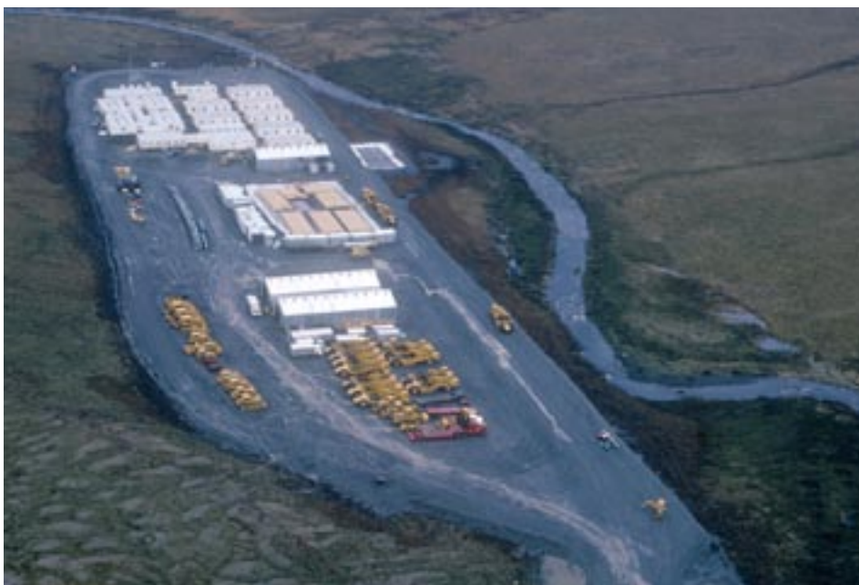
A Happy Valley Camp, 1970, one of 29 camps needed to build the oil pipeline. Construction camps required for a new gasline will use previous camp locations whenever possible.
