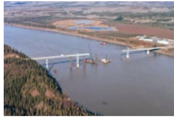
The Yukon River Bridge was completed in 1975. It is unlikely a gas pipeline will be able to share this bridge for a variety of reasons.
