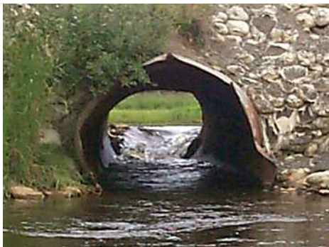
Undersized and eroded culverts blocked fish passage at Squaw Creek. Replacing them opened up 15 miles of habitat.
