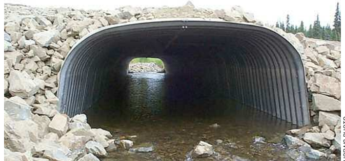
Undersized and eroded culverts blocked fish passage at Squaw Creek. Replacing them opened up 15 miles of habitat.
