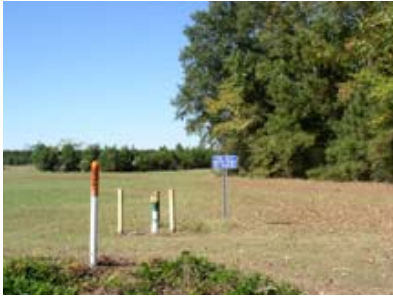
All the dry hydrants were clearly marked for easy identification during an emergency.
