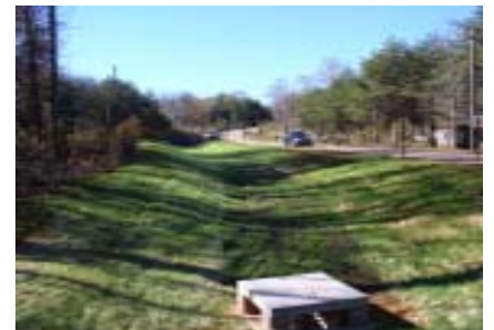
Ridge Road after filling in the gully.
